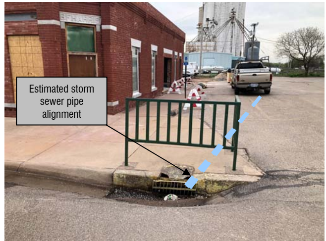
219 W. Main (photo taken during the Empire Taco building remodel in 2019)
