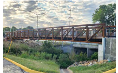
10 th Street Bridge Topeka, KS
