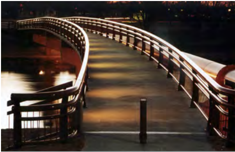
Pedestrian Bridge over the Arkansas River Wichita, KS
